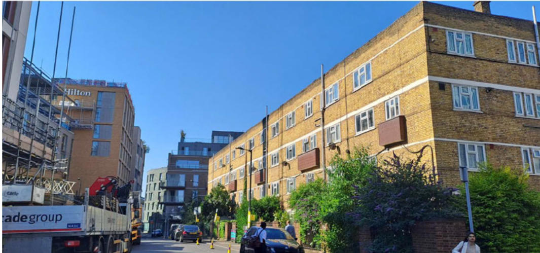
View showing Friars Close on the right and the Hilton Hotel and associated extension on the left.
