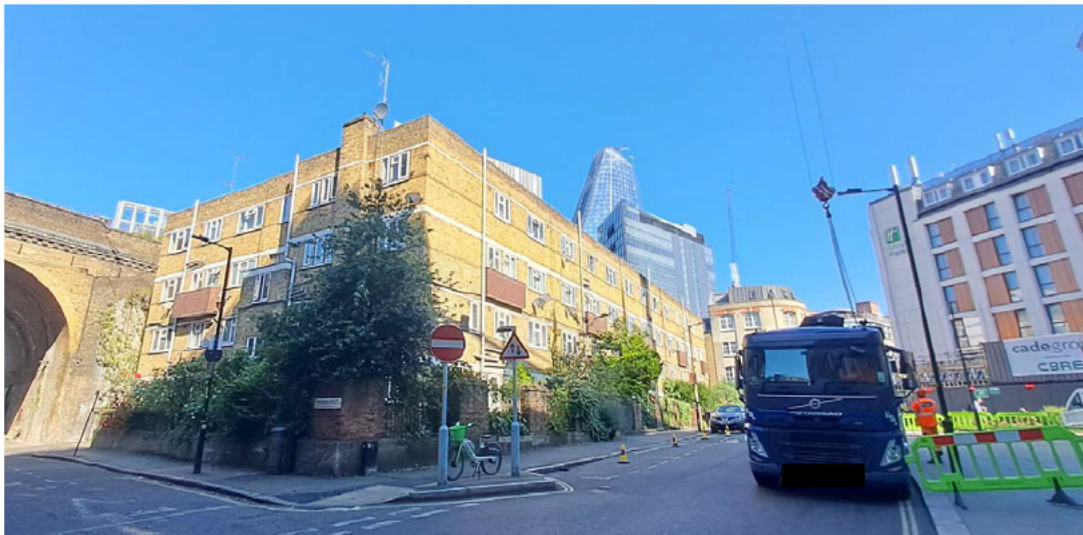
View showing Friars Close with One Blackfriars shown in the background.
